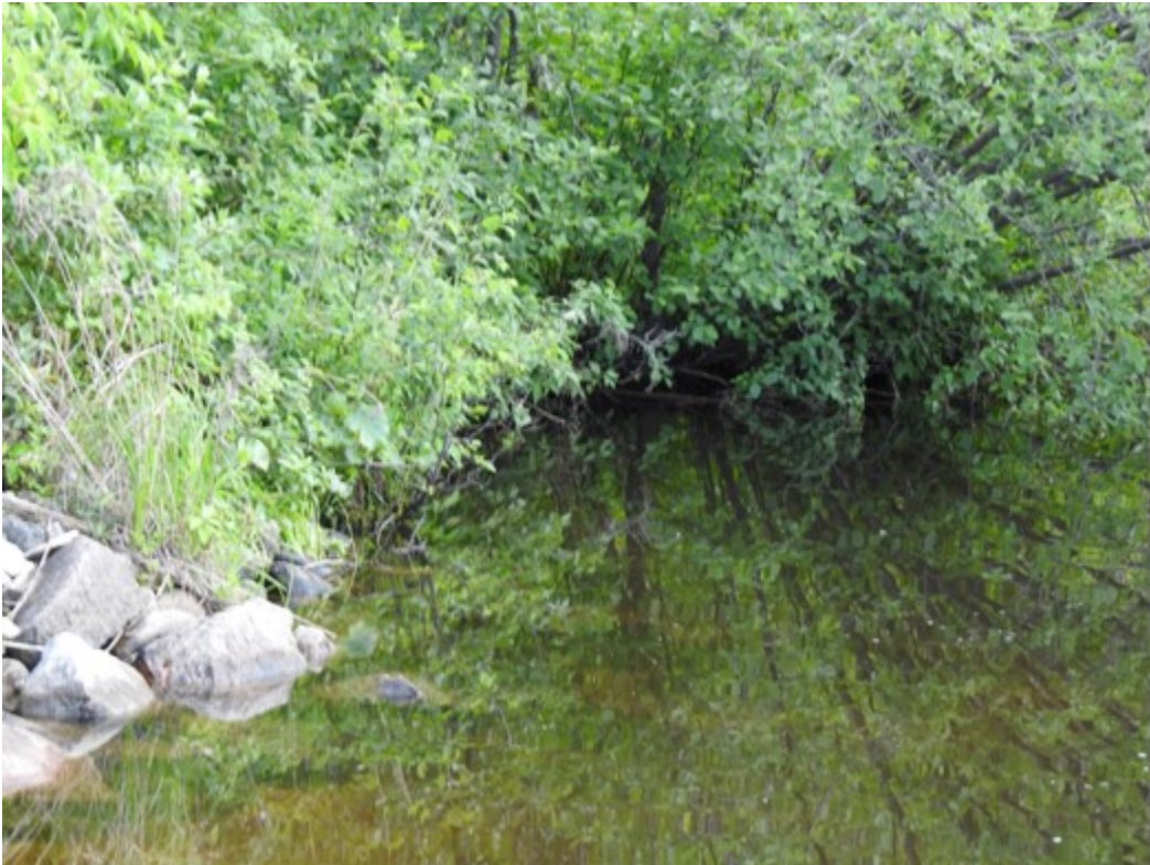
Pictures 7, 8, 9, 10 are of our property shoreline Picture 1 shows the amount of shoreline that has been washed away in approximately 5 years if it is not rocked. Even rocking the shore needs to be repaired every year with new rock. Even the rock gets moved and washed away from the boat traffic. The shoreline trees are dying and falling in. Every year more is washed away from wake boats and ski boats turning in front of our property to avoid the congested boat traffic going around the island. We need a No Wake zone right here for both reasons safety of peoples lives, as well as the massive erosion happening
